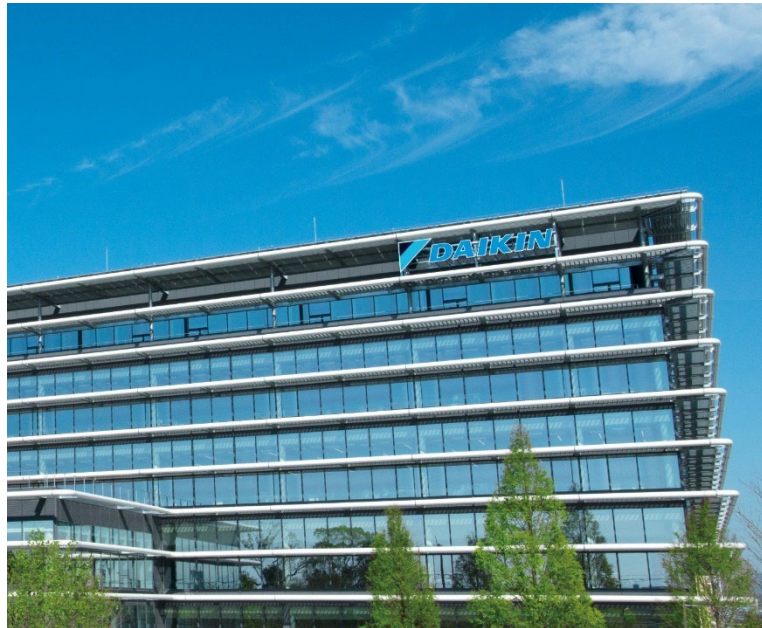
Daikin Technology Innovation Center
