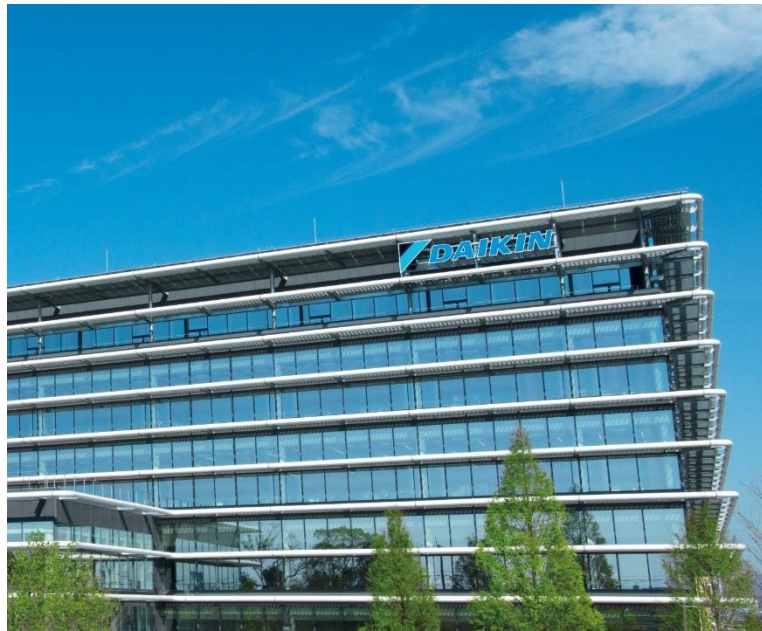
Daikin Technology Innovation Center
