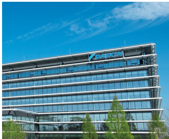
Daikin Technology Innovation Center
