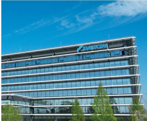
Daikin Technology Innovation Center
