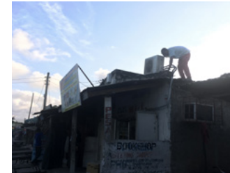
Installing an outdoor unit on a house
